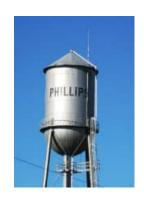
The City of Phillips storage facilities consist of two above ground, elevated tanks or water towers. One water tower is located on Peterson Drive. The above ground tank is able to hold 100,000 gallons of water. The second water tower is located at Balsam Street. The tank can hold 250,000 gallons of water.
